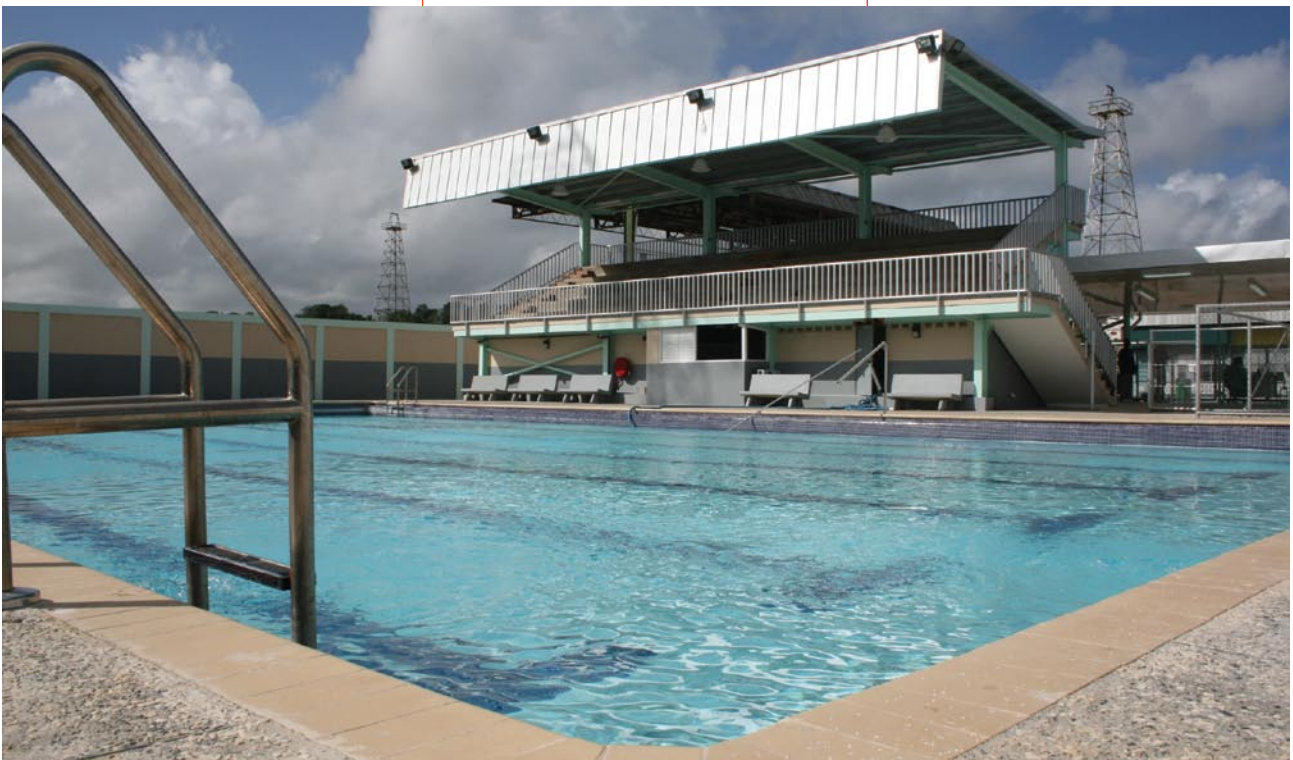
The swimming pool was constructed at the Southwest Regional Sporting facility, Coronation Park, Egypt Village.
