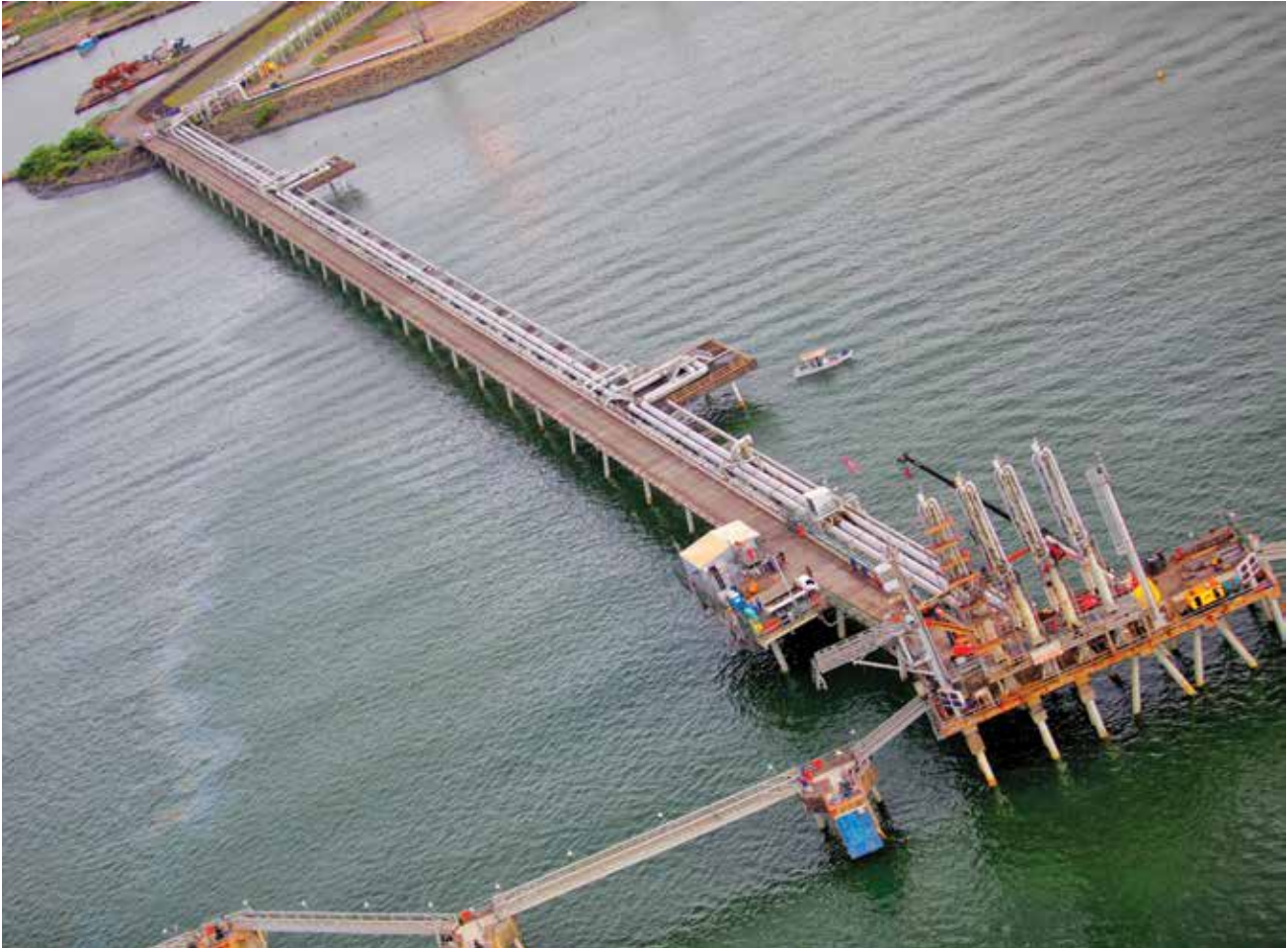
Aerial view of Atlantic's loading arms which allow for the transfer of LNG to LNG vessels
