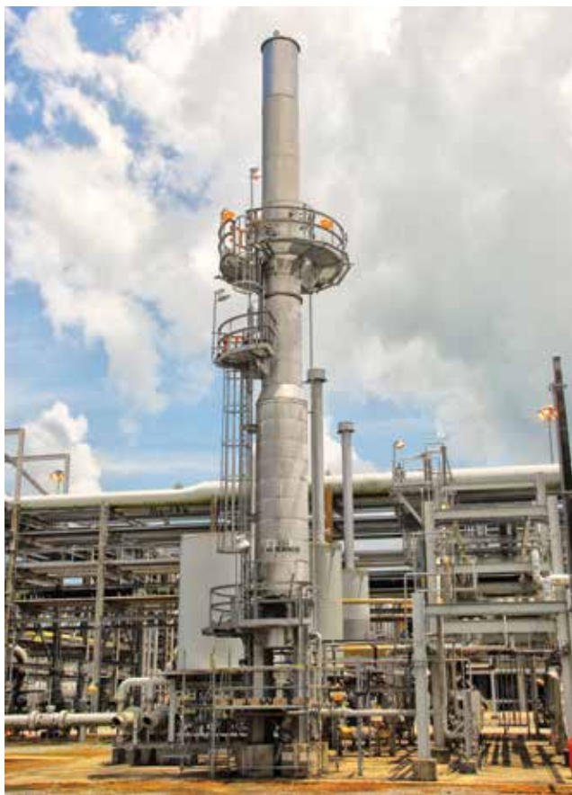
Acid Gas Incinerators on Train 3
